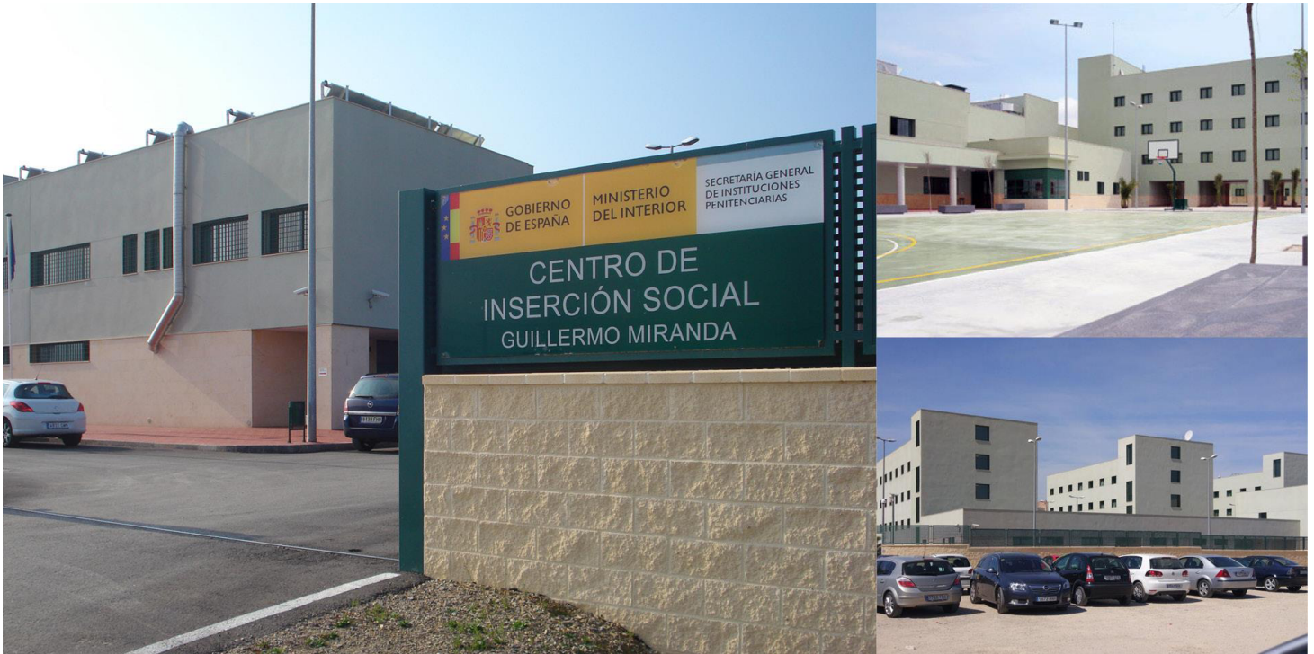
reinforcement concrete structure
